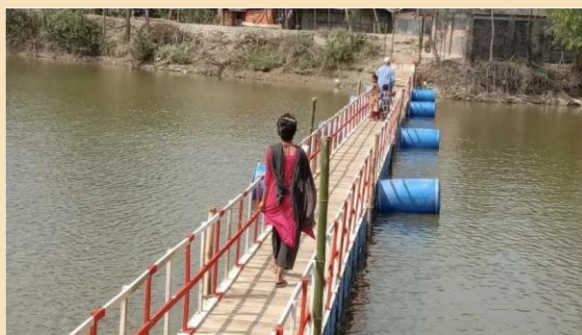
Photo: The Koyra Floating Bridge in use over the Patharkhali Canal
